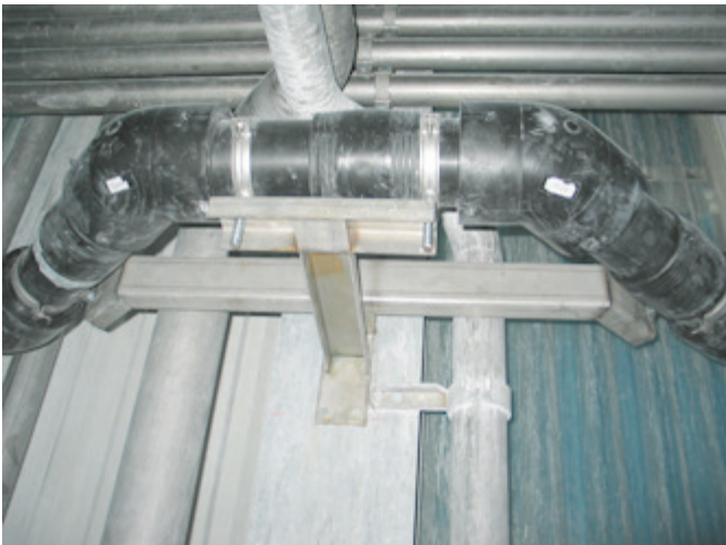
Double containment system fixed point
